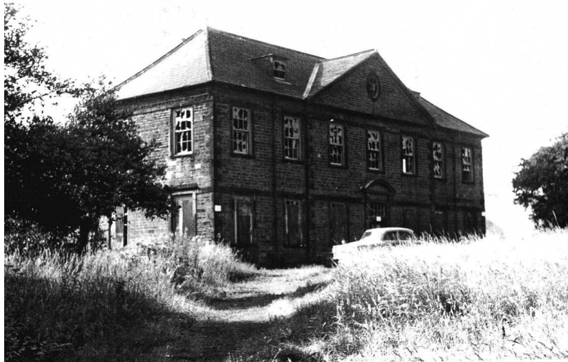
Netherwood Hall in 1963, shortly before its demolition
